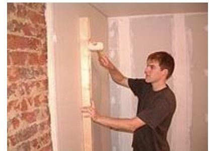
(Foto: Recticel Insulation)
