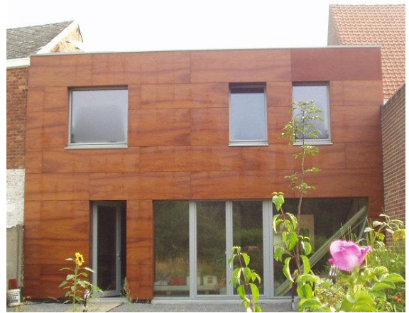
Multiplexplaten (Bruynzeel) (arch. denc!-studio, Gent)
