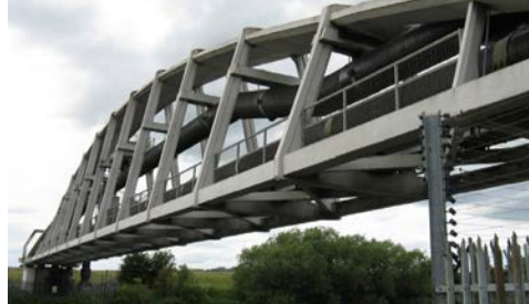
Peston Pipe Bridge - Ingleby Barwick (UK)
